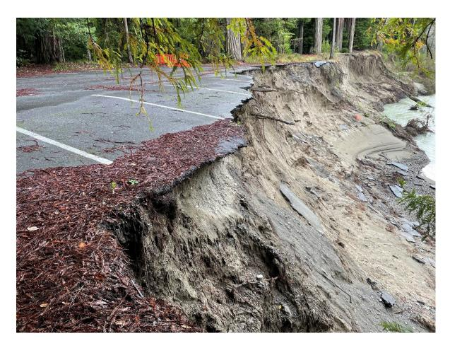
The photo above shows the embankment slope failure at California Federation of Women's Clubs Grove Day-use parking lot. Embankment instabilities including cracks, slides, and depressions are a result of the natural impacts of extreme weather, including heavy rainfall and flooding events.
